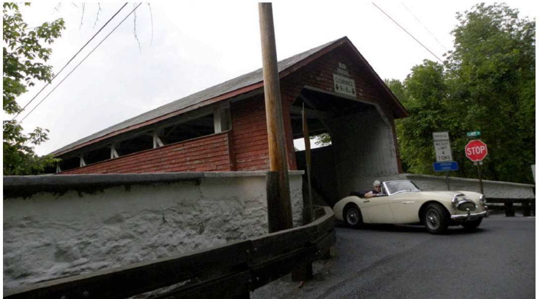
Gerry and E.J. Kunkle crossing one of the bridges.
