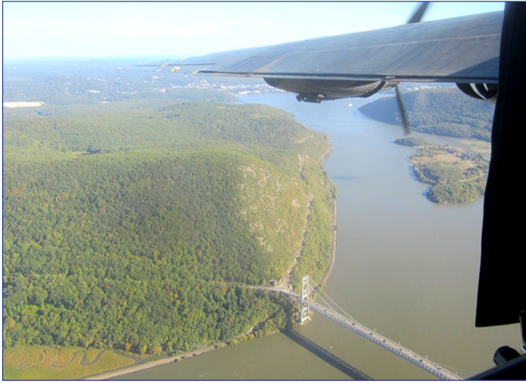
Bear Mountain Bridge
