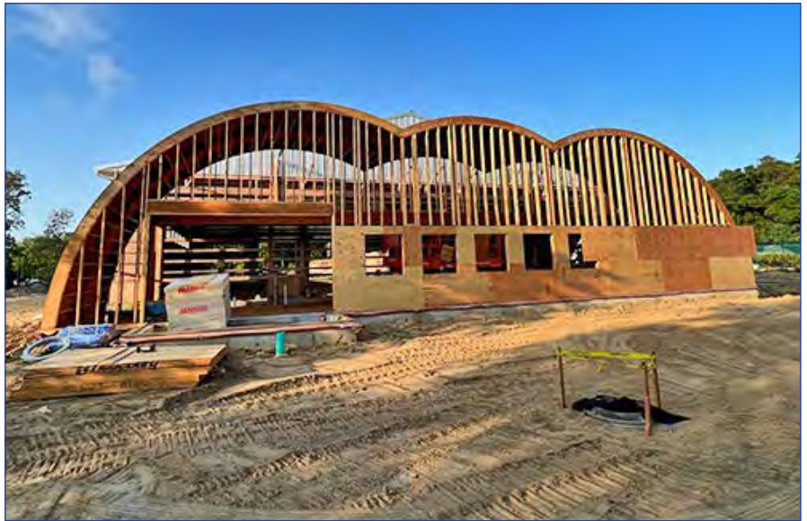
New framing of the front.
