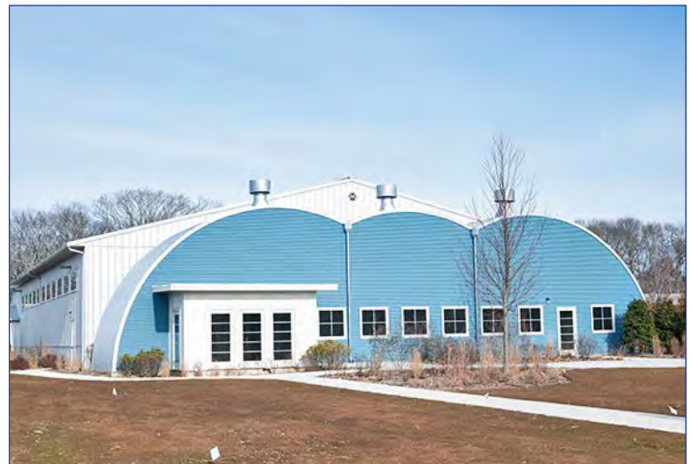
New facade in the style of the old museum.
