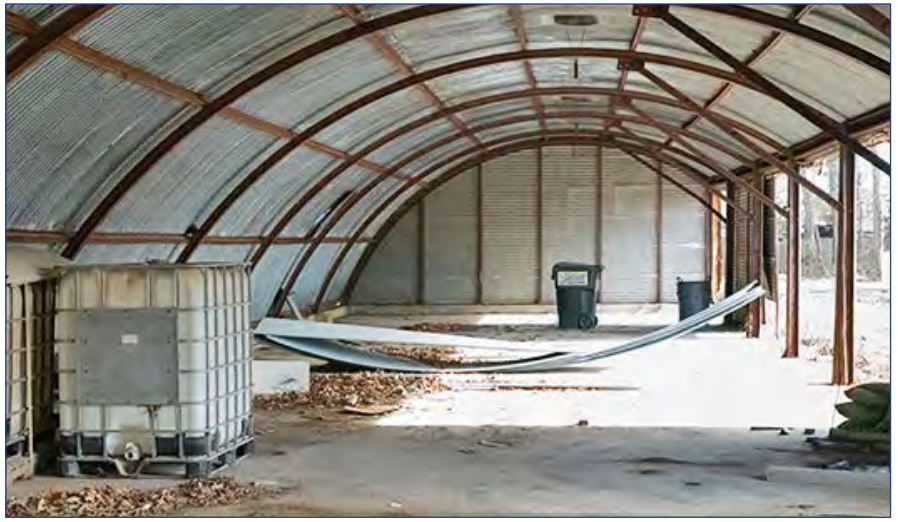
Interior of old outbuilding shows Quonset hut construction.
